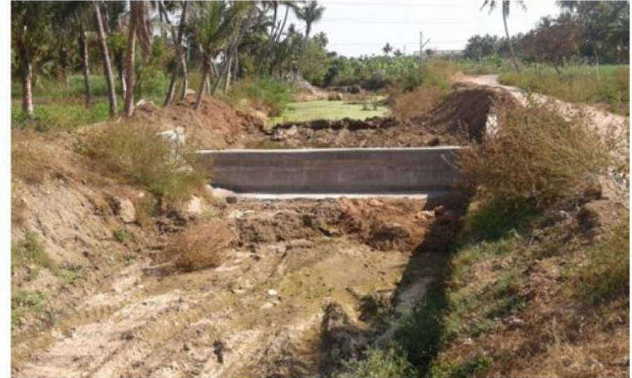
New Check Dam in without Water
