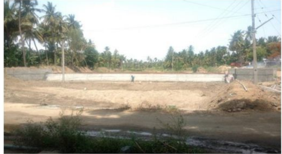
After New Check Dam Construction Without Water
