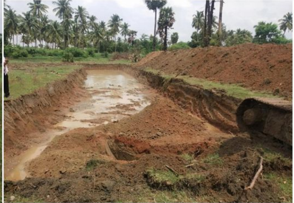
During the Work
