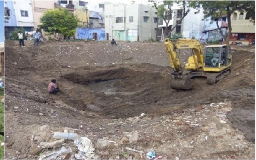
After Deepening Work
